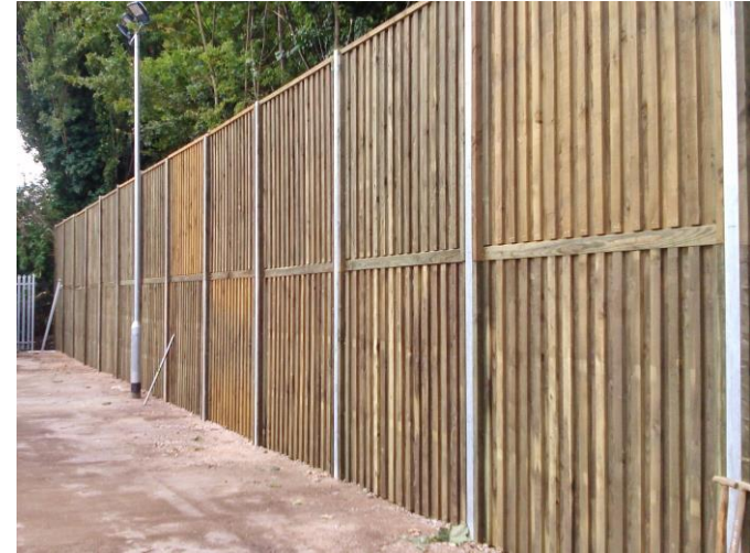
Proposed treatment to be fixed in front of existing boundary to mitigate noise and visual impart to both the development and the railway line. See detail.
