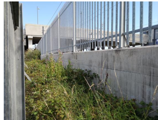
4. The existing Railway Boundary at Proposed Block 17 also to be retained.
